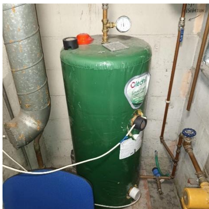
Photo 1 & 2 - view of 200 litre electric calorifier (HWS01) located in 2 nd floor boiler room with temperature gauge showing unsatisfactory operating temperature of water heater.
