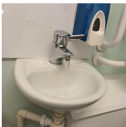
Photo 5 & 6 - view of typical thermostatic mixing tap (TMT) with associated strainers.
