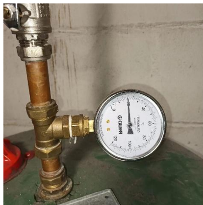
Photo 1 & 2 - view of 200 litre electric calorifier (HWS01) located in 2 nd floor boiler room with temperature gauge showing unsatisfactory operating temperature of water heater.
