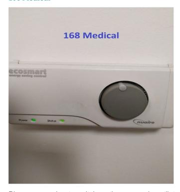
Please remember to switch on the powered ventilator an put it on **full speed** before directing the patient to the isolation room by the host. The clinician should switch it off after cleaning the room, once the patient has departed.
