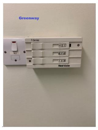
Please remember to switch on the powered ventilator an put it on **fan speed 3** before directing the patient to the isolation room by the host. The clinician should switch it off after cleaning the room, once the patient has departed.
